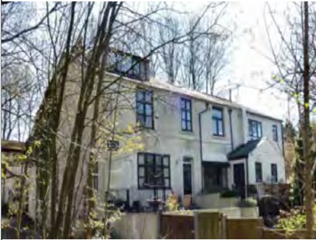
This was originally a workhouse in Royton. It has since been rebuilt.
